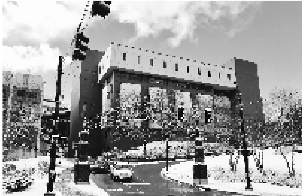
BEHIND THE SCENES -- Duquesne facilities management is responsible for making sure campus is well-maintained for students -- MEGAN KLINEFELTER/STAFF PHOTOGRAPHER
